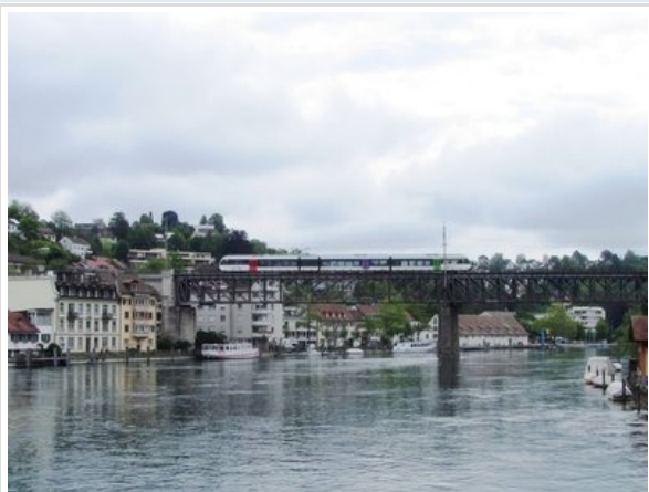
Schaffhausen, Rhine Bridge, 10.06.19
