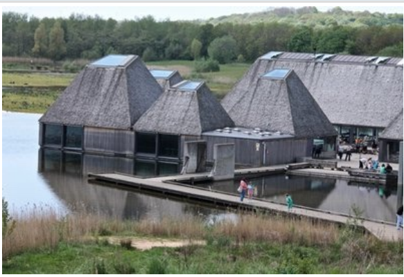
Brockholes Floating Restaurant
